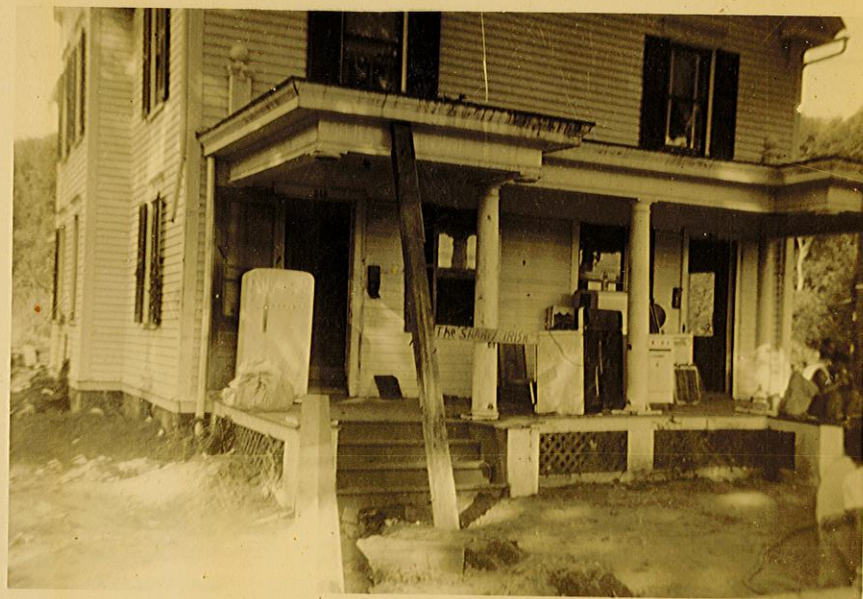
McManama left / Rherr right None of items on porch and in yards were useable.
